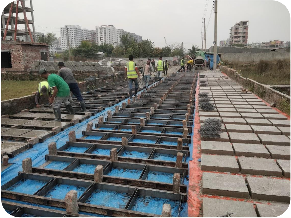
DPDC Underground Cable Line Slab Casting, Dhaka.
