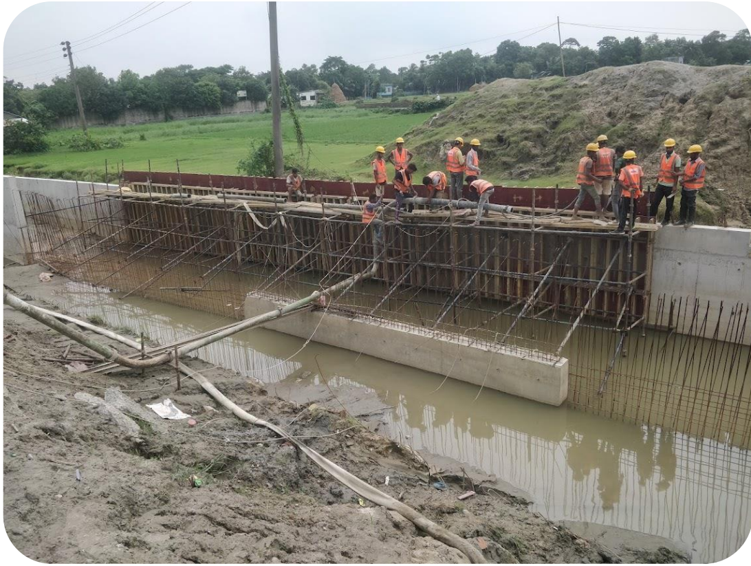
RCC U Drain Works at Brahmanbaria
