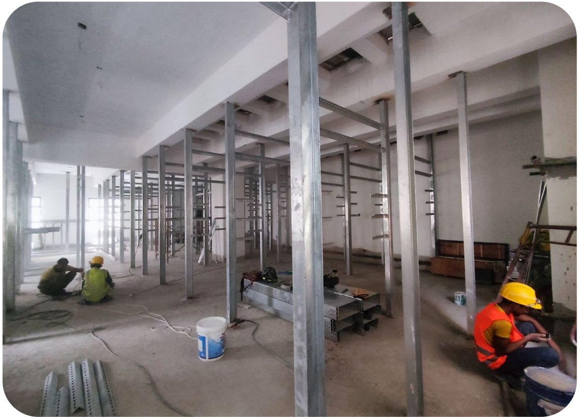
Sub-Station Steel Structure Work at Basila, Dhaka.
