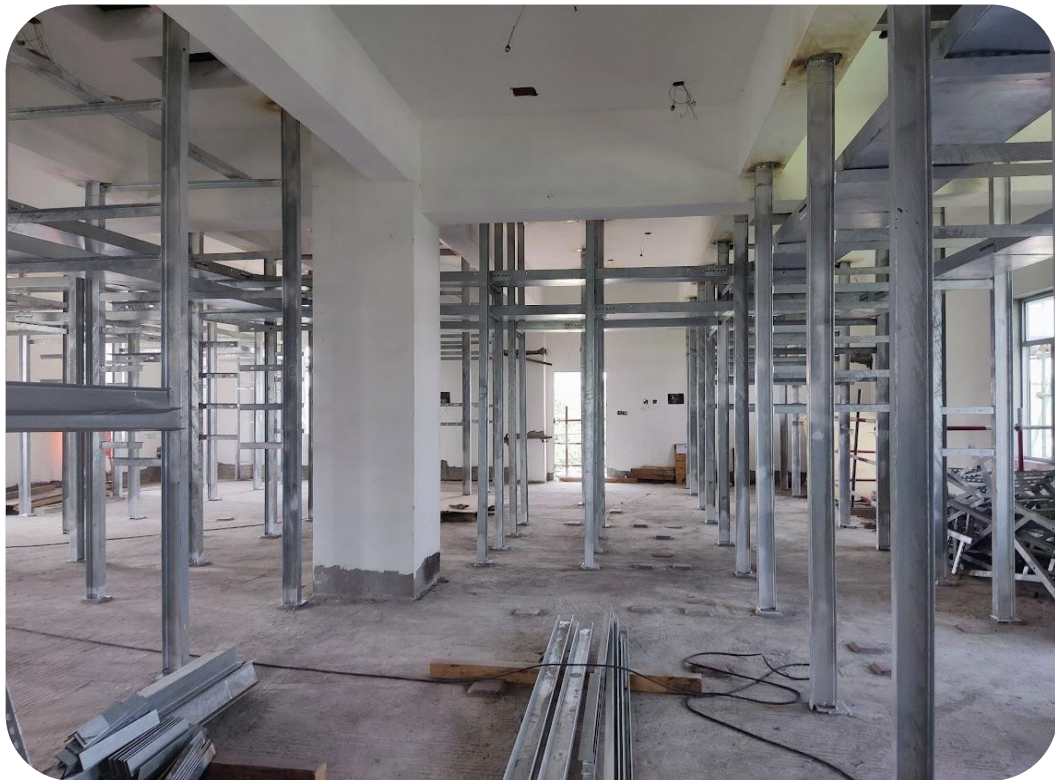
DPDC Sub-Station Project at Shyamoli, Dhaka.
