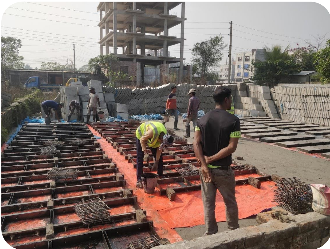
DPDC Underground Cable Line Slab Casting, Dhaka.
