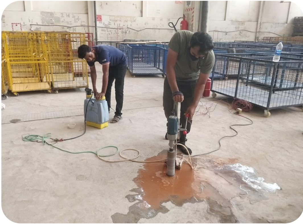
Core Cutting Work at Daraz Bangladesh Wirehouse, Tejgaon, Dhaka.
