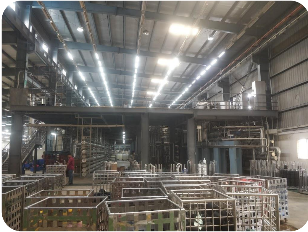
Mezzanine Floor Work at Mawna, Gazipur.
